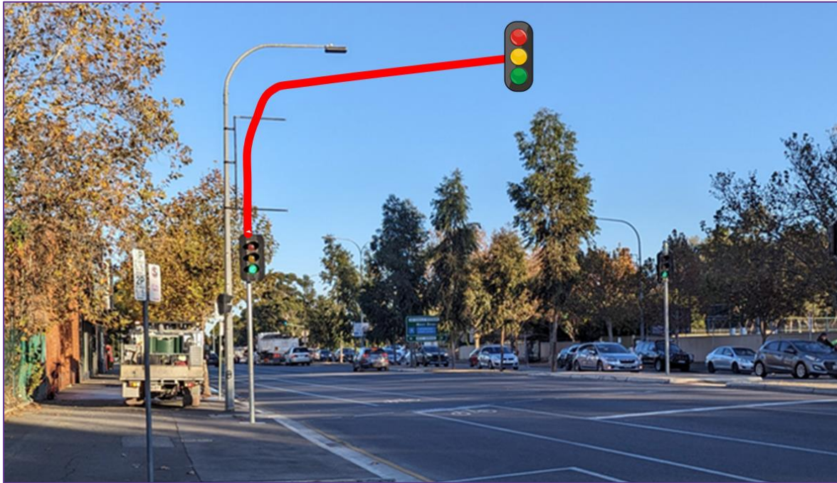
Figure 4.1 Install Overhead Mast Arm at the Signalised Crossing
